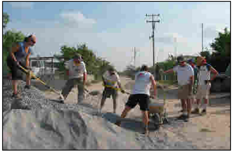
shifting sand and gravel to the cement-mixing pit
